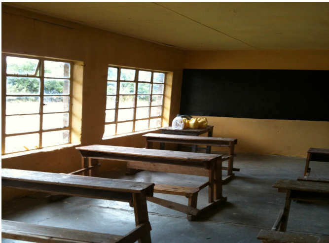
With new windows in place of the metal sheets the light pours into the classroom creating a much better working environment.
