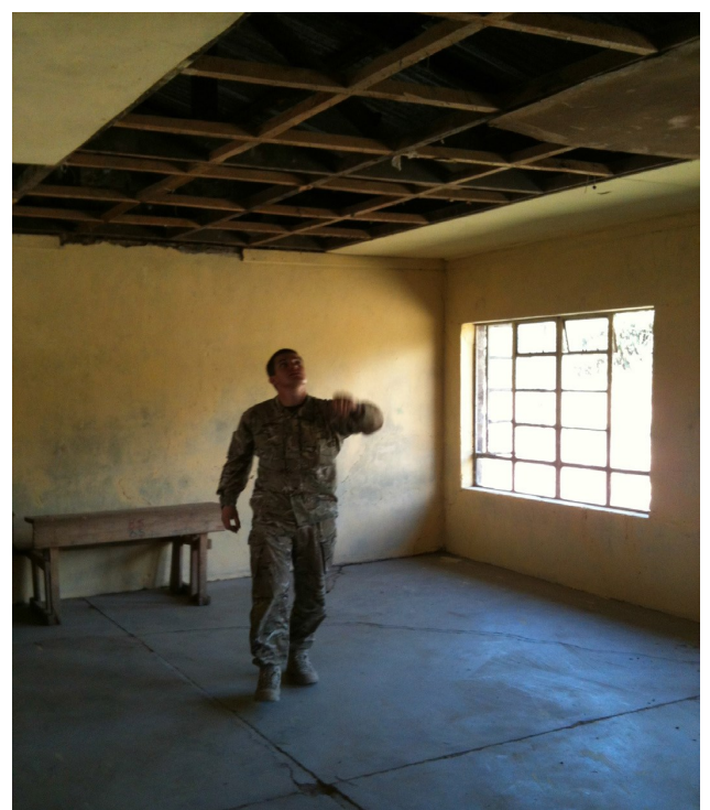
Cpl Bradshaw assesses the work required on the ceiling (right)
