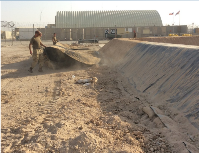
Last Bundliner Removed
